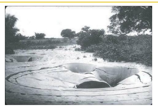
Fig. 5: Liquefaction during the earthquake (Source: archives.assam.gov.in)
